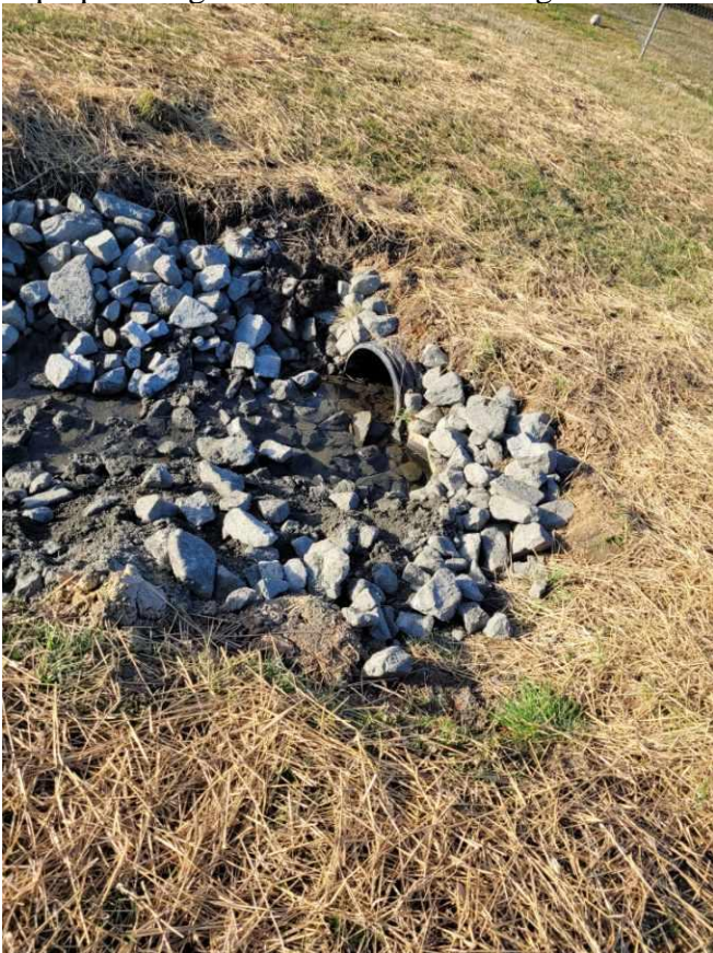
Riprap at fairgrounds for storm drainage
