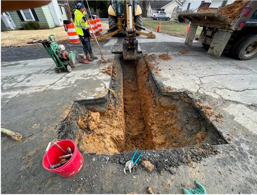
Charles Street Leak repair
