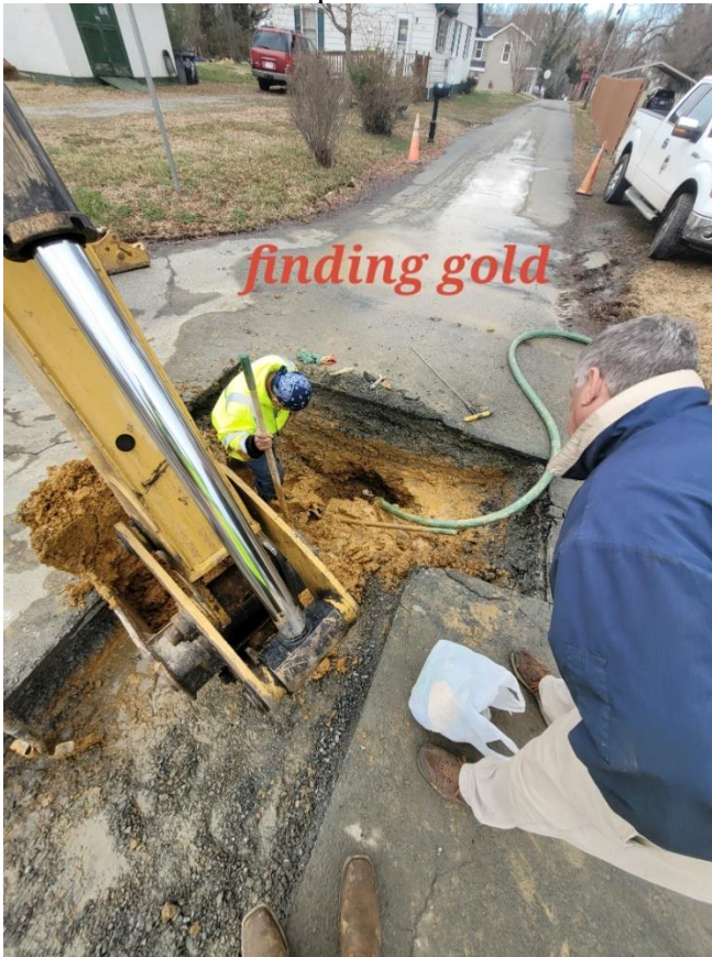
Charles Street Leak repair
