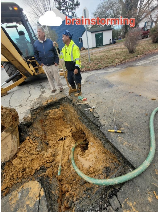
Charles Street Leak repair
